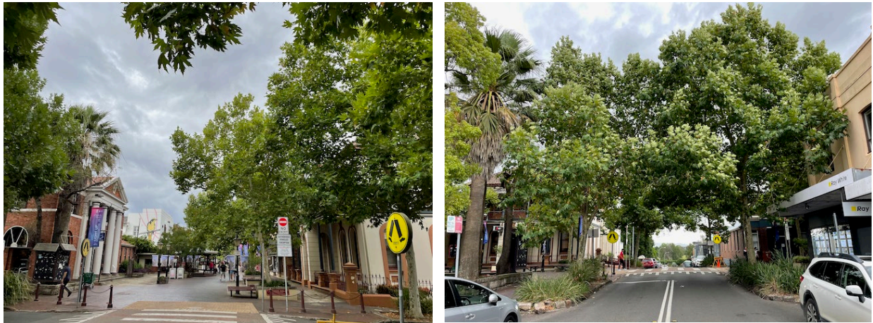
Figure 5. Services are now underground in Windsor town centre.
